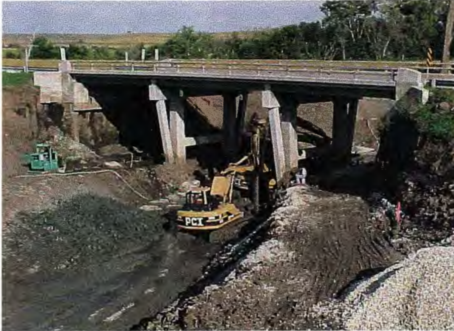
Figure 12. Project site looking north-east during pier installation
